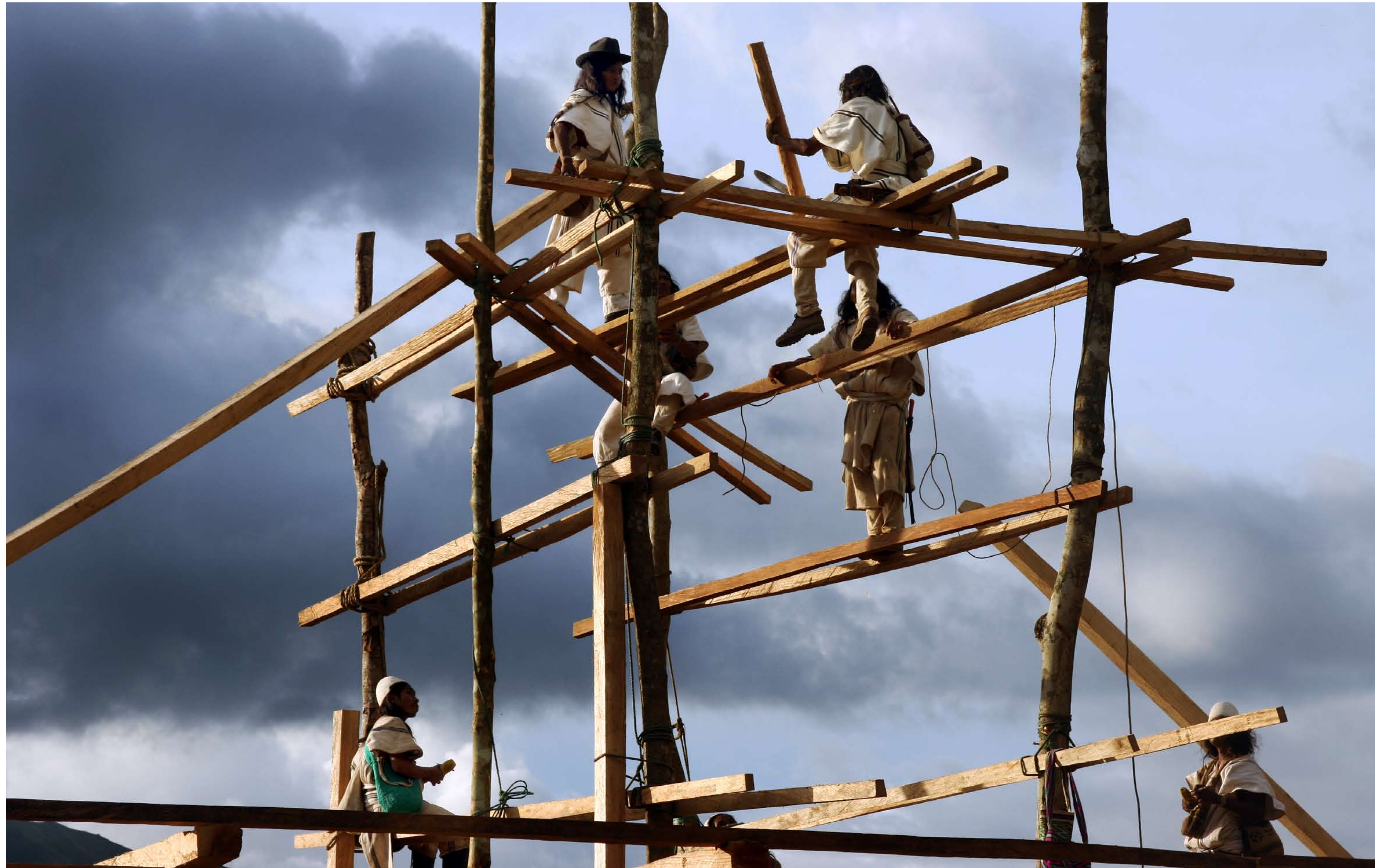
Arhuacos building a house
