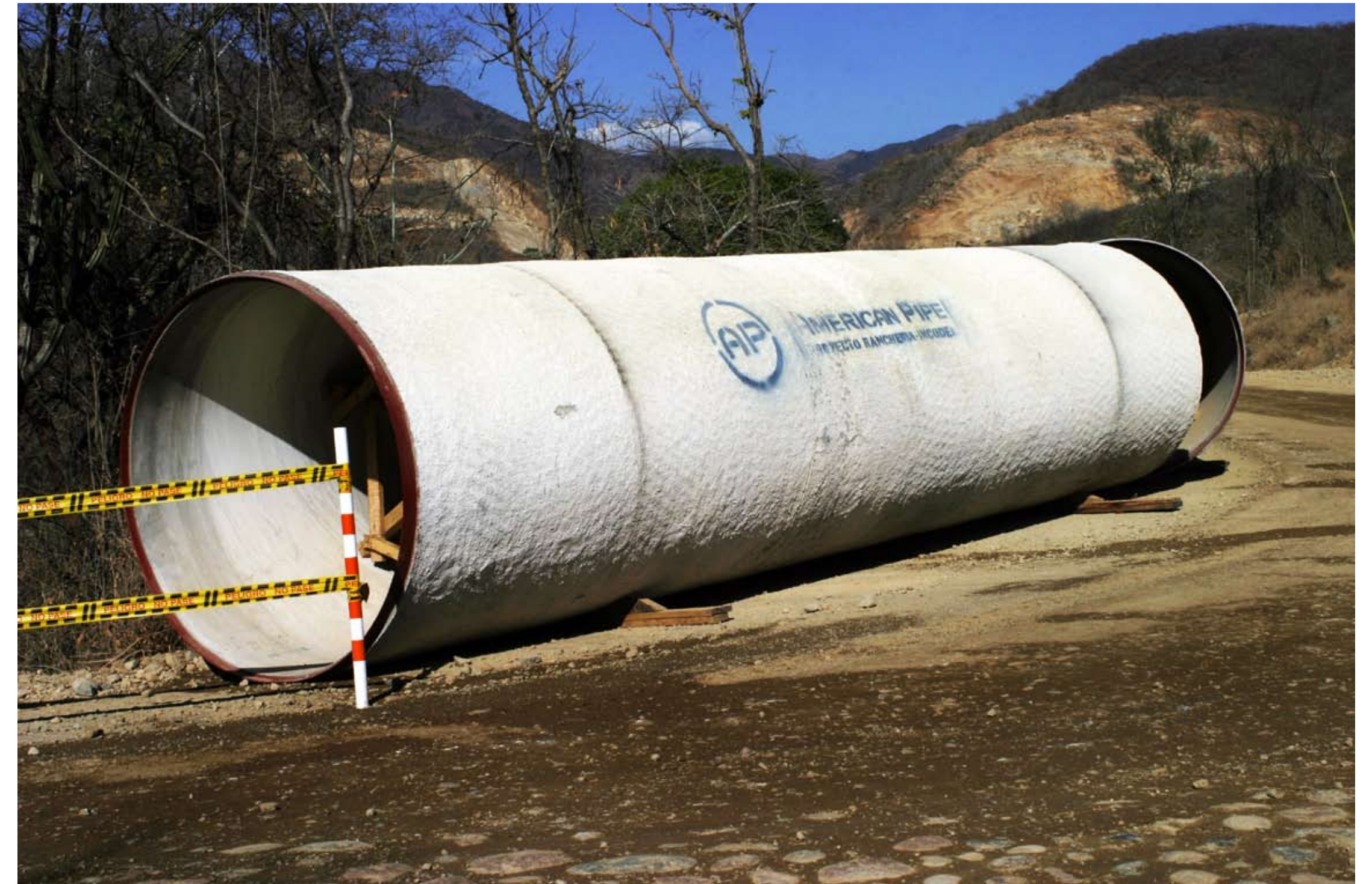
Huge Dam construction at the Ranchería Sacre River
